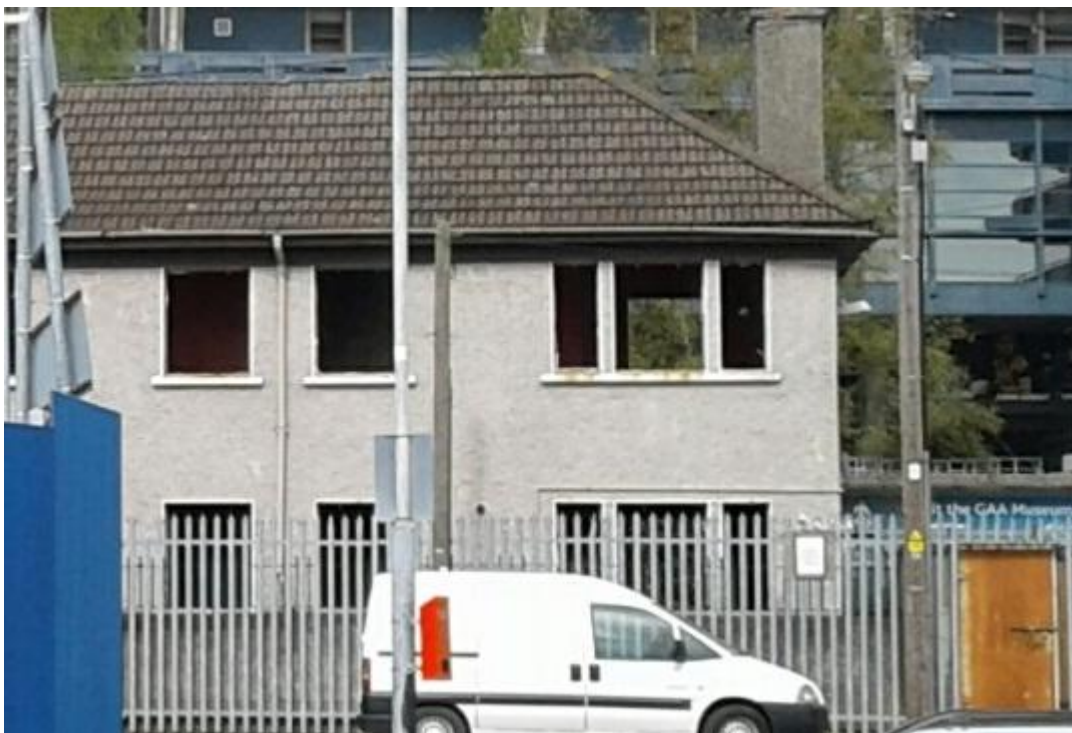
Demolition contractor now on site at Saint Andrews Court.
